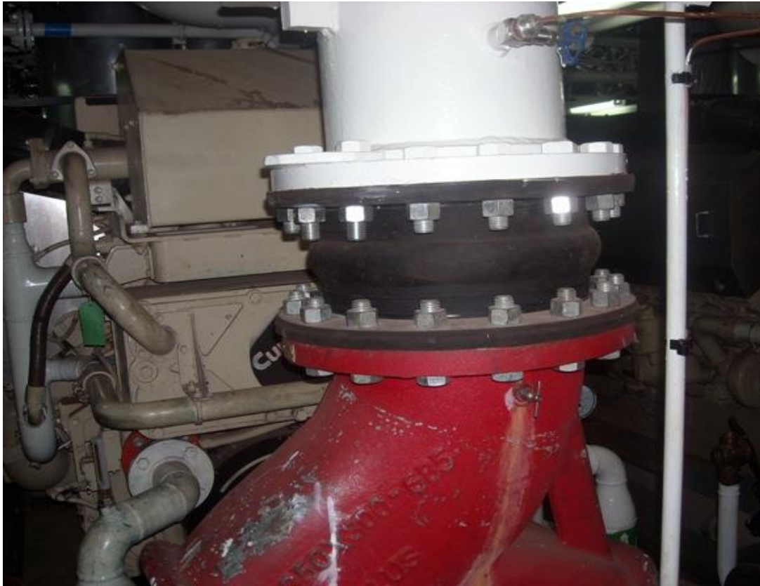
Fig. 1: Expansion Joint with corrugated bellows
